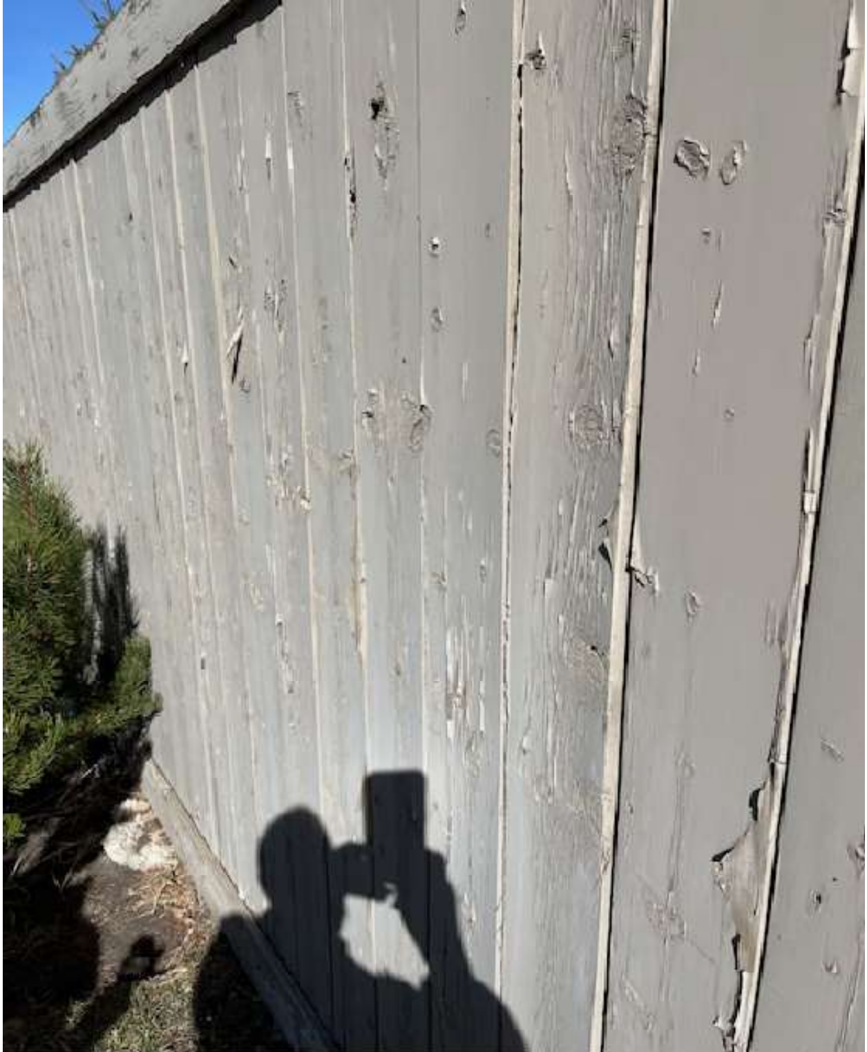
Figure 15 stain/paint peeling
