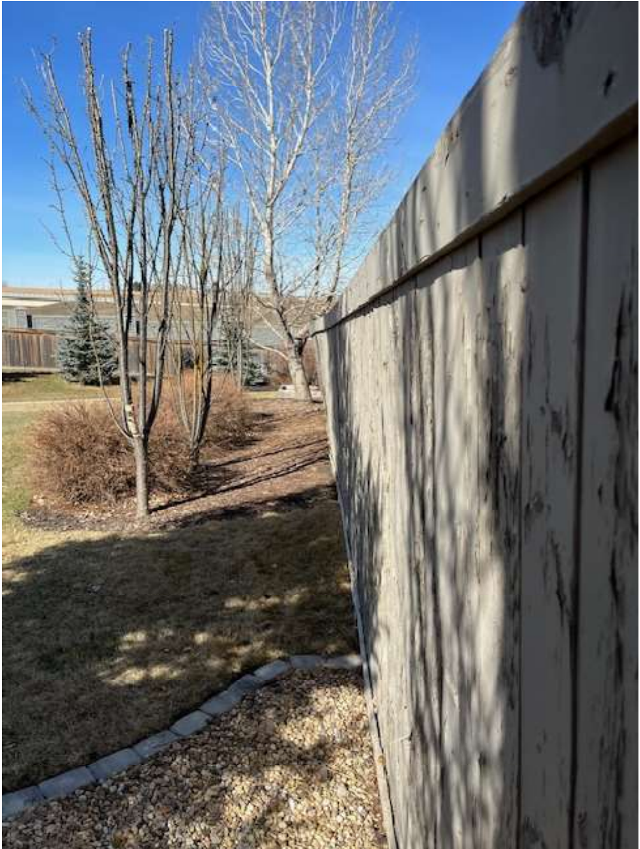
Figure 20 note the bow in the fence and deteriorating boards
