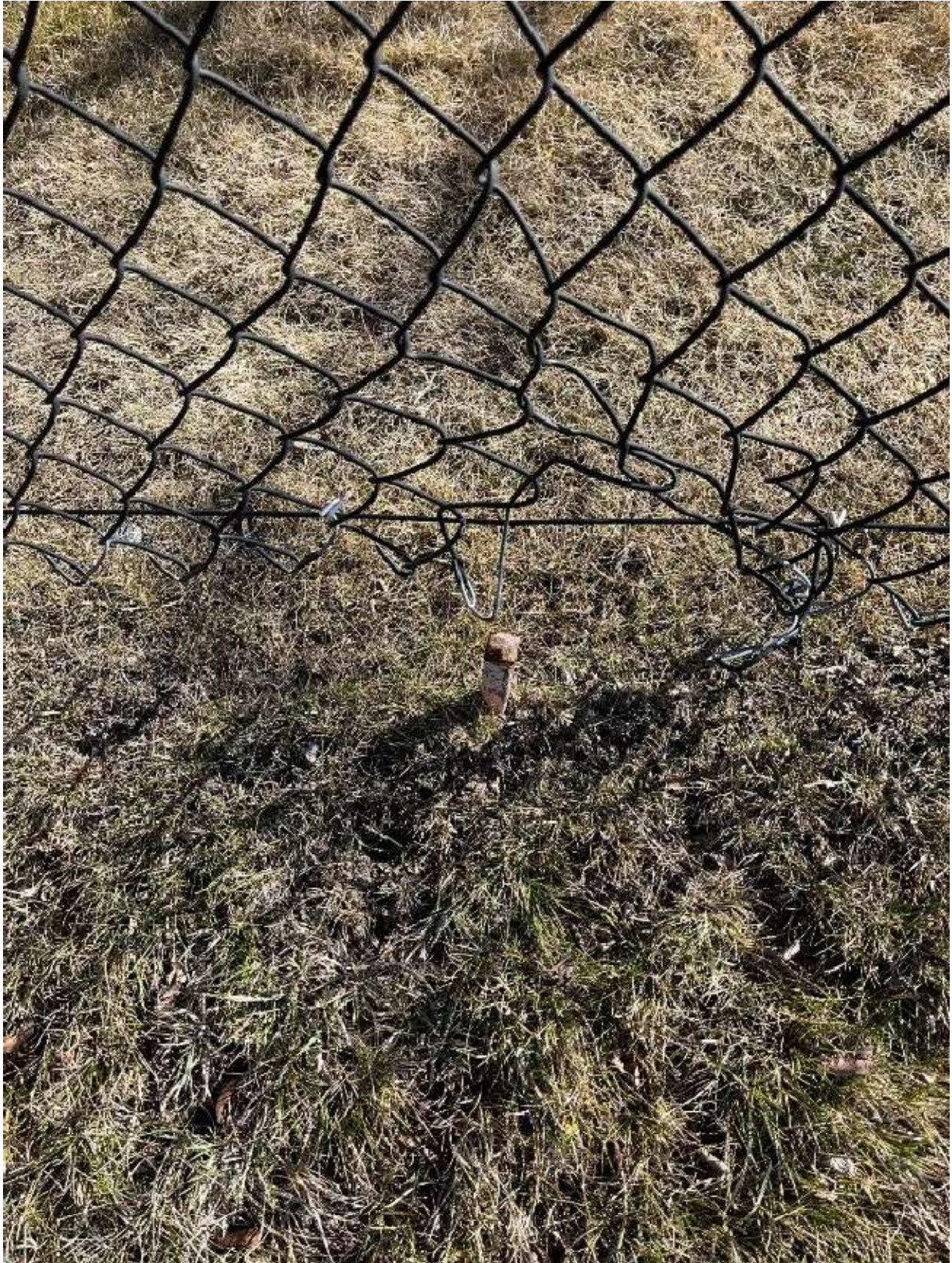
Figure 8 Chain link indicating separation
