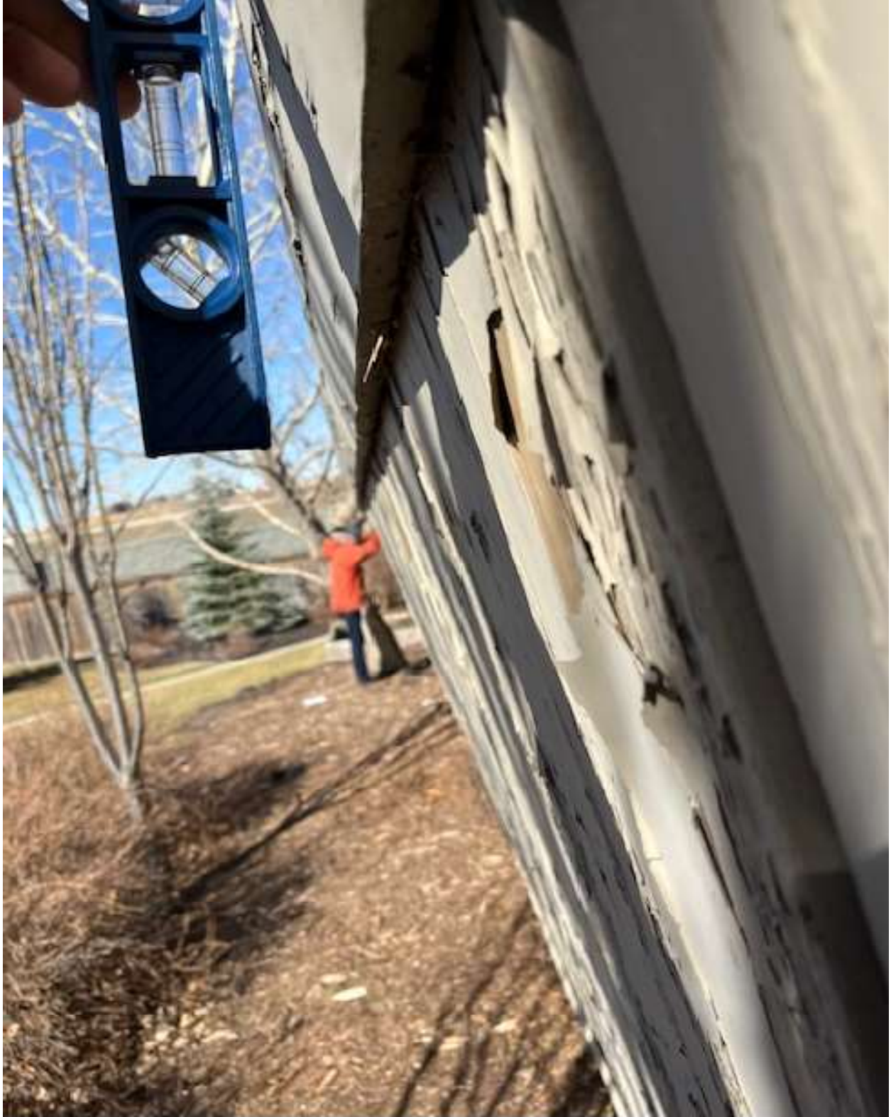
Figure 17 Fence leaning at least 20 degrees
