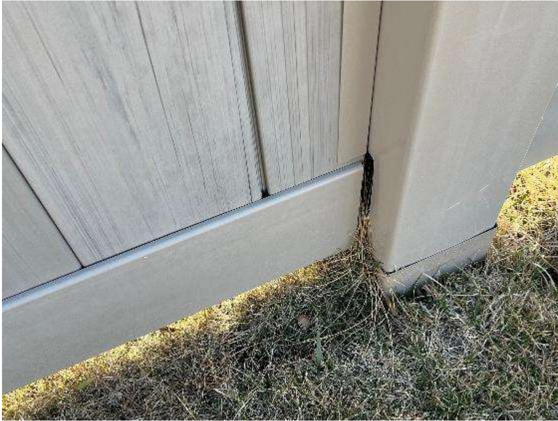
Figure 2 Vinyl fence with bottom rail adrift of the post, and easy fix to simply position it back in the post
