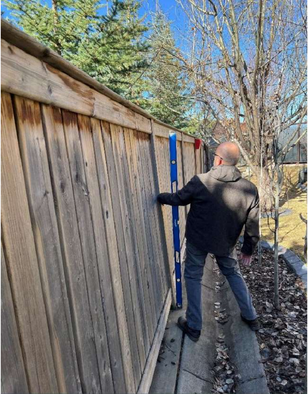
Figure 30 the south perimeter fence showing the lean to the south. The posts are embedded in concrete rendering the fix to vertical a relatively expensive task.
