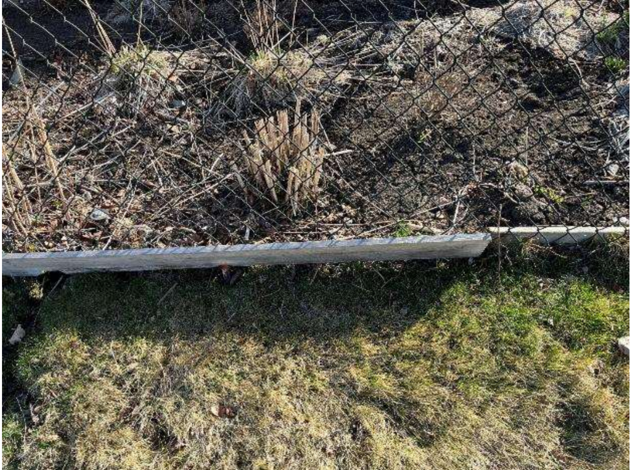
Figure 5 Chain link fence showing material piled against the fence placing extra load on the wire stringer and chain links
