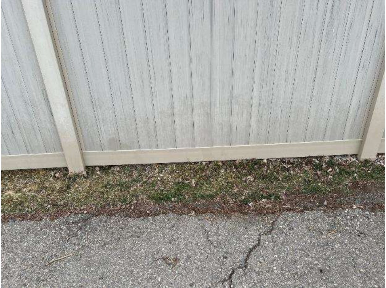
Figure 3 Vinyl fence along 24 St showing staining mainly due to snow removal with a blower piling snow against the fence.
