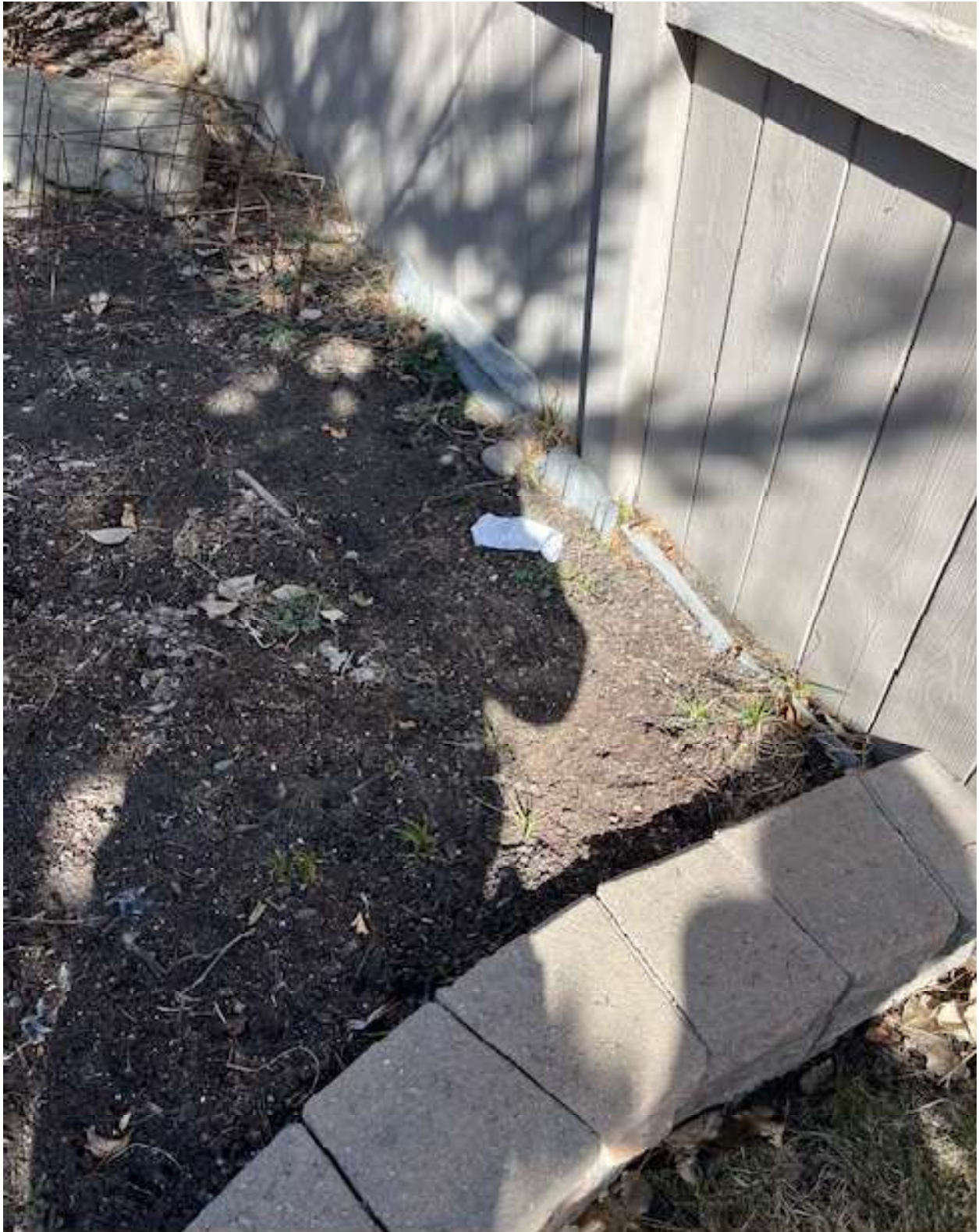
Figure 12 an example of material piled next to the fence retaining moisture and accelerating decay of the wooden rail and boards
