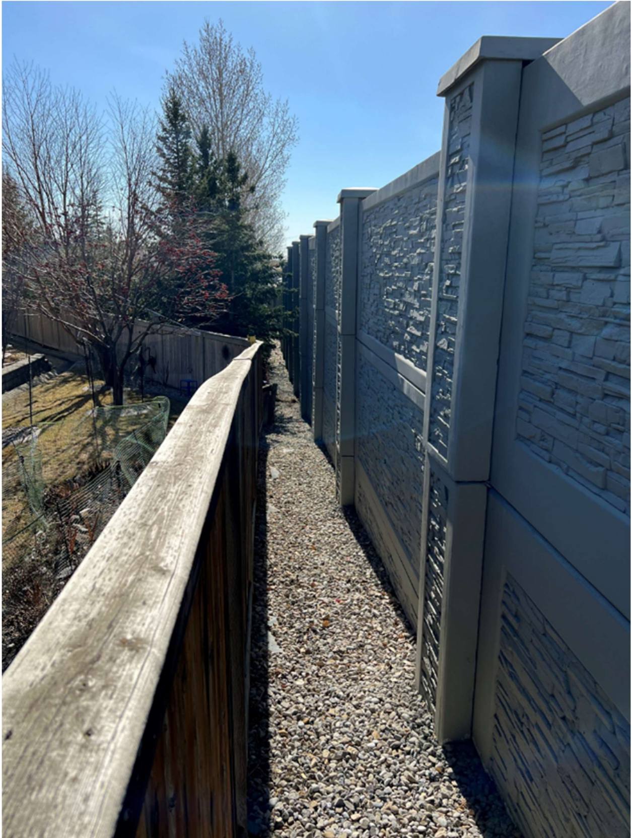
Figure 24 Second view of the gap between the west perimeter fence and sound barrier; note the intact condition of the top plate.
