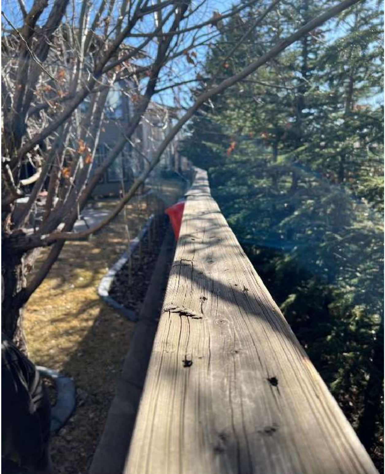
Figure 31 South perimeter fence indicating a top plate in good condition and the non-bow to the south.
