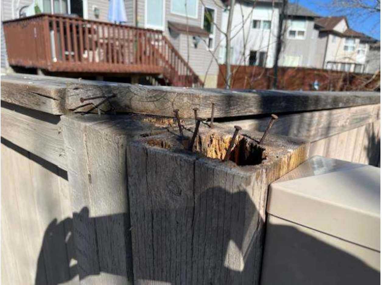
Figure 13 Post cap missing accelerating decay of the post.
