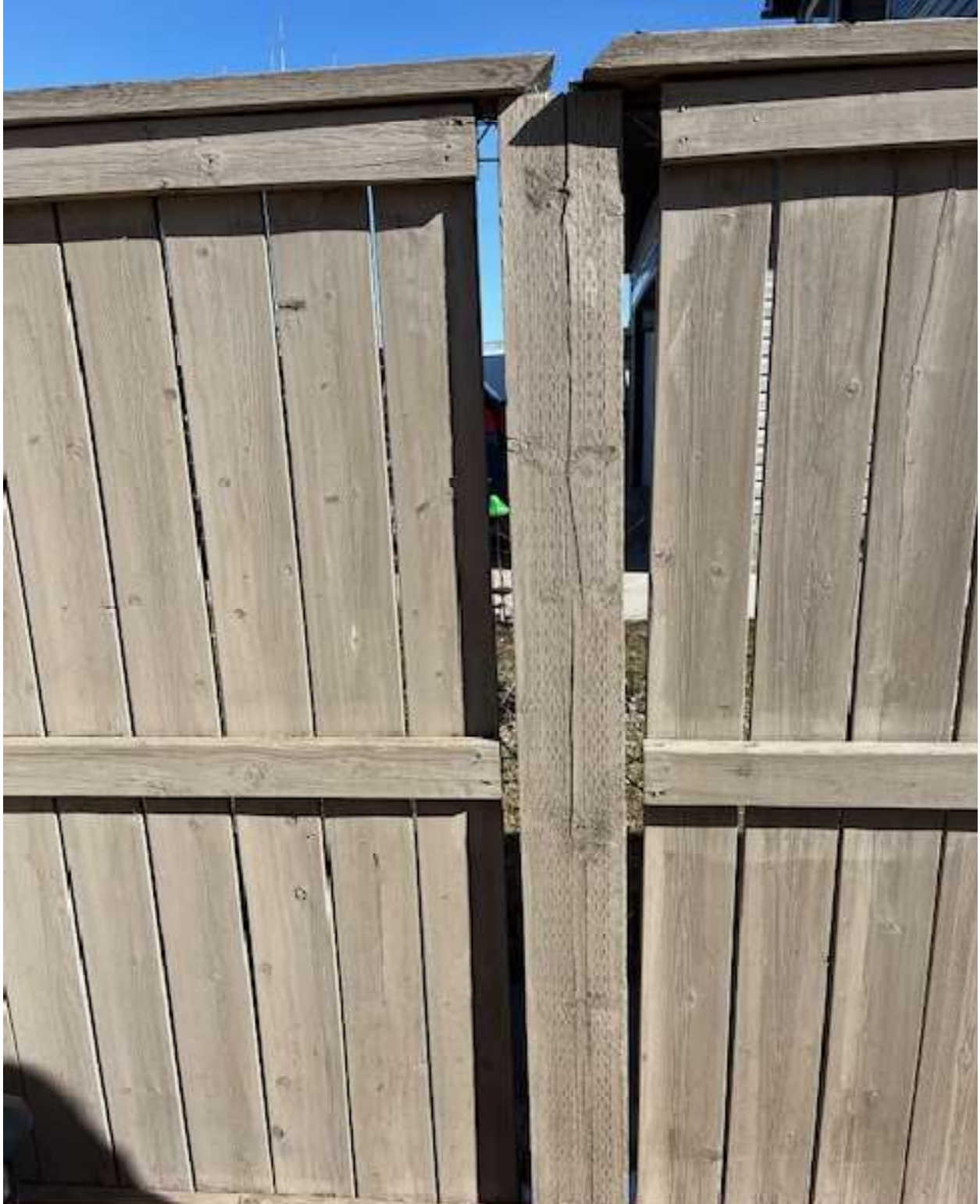
Figure 14 fence components separating from the post.
