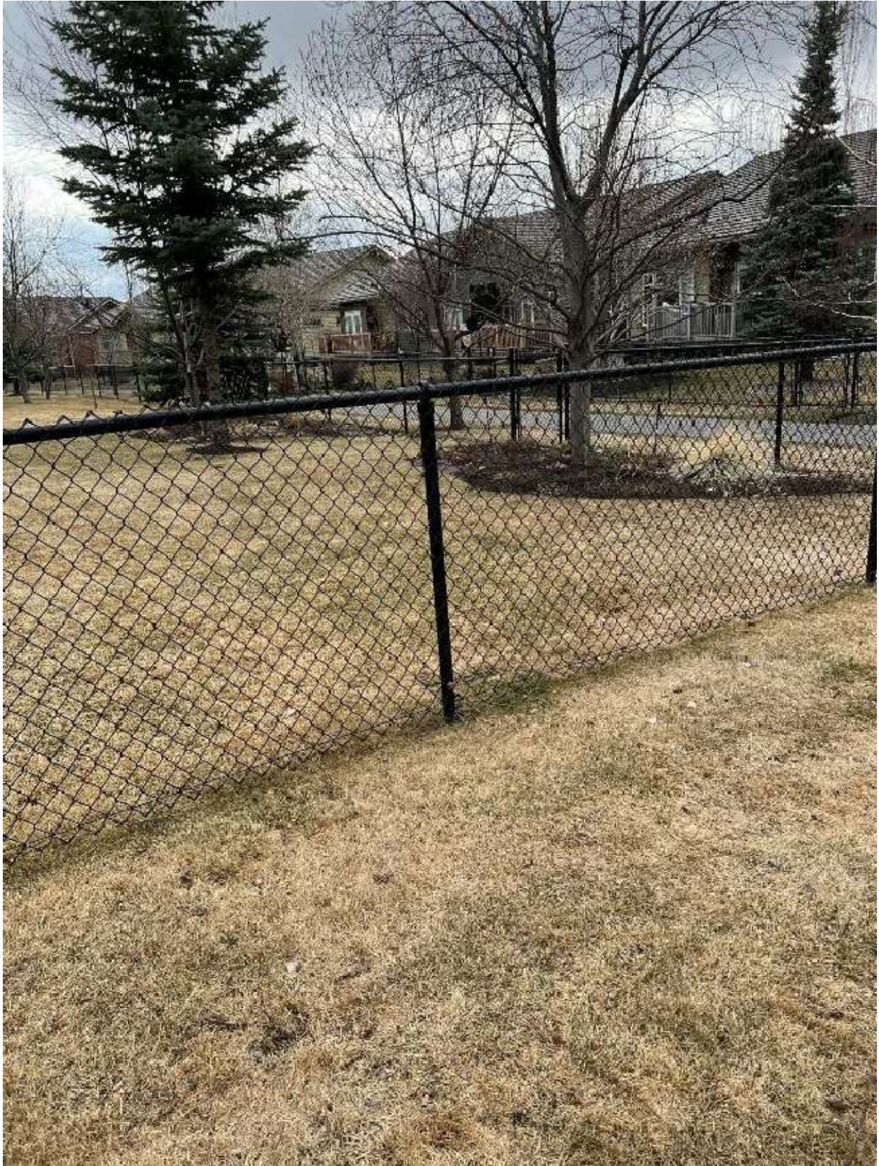
Figure 10 Chain link fence as it should be, no loading on the bottom stringer and chain links.
