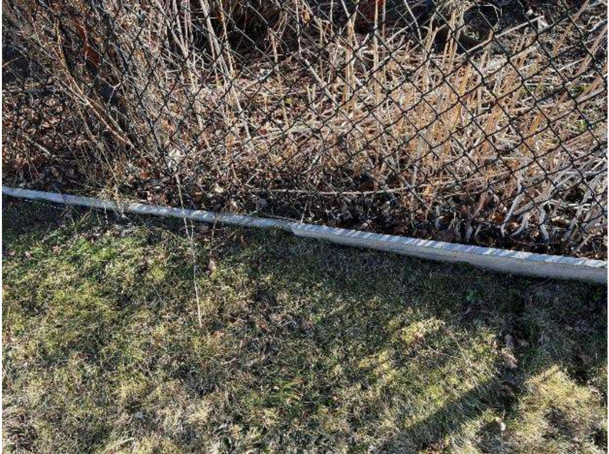
Figure 6 Chain link fence showing typical material loading the wiring stringer and chain links
