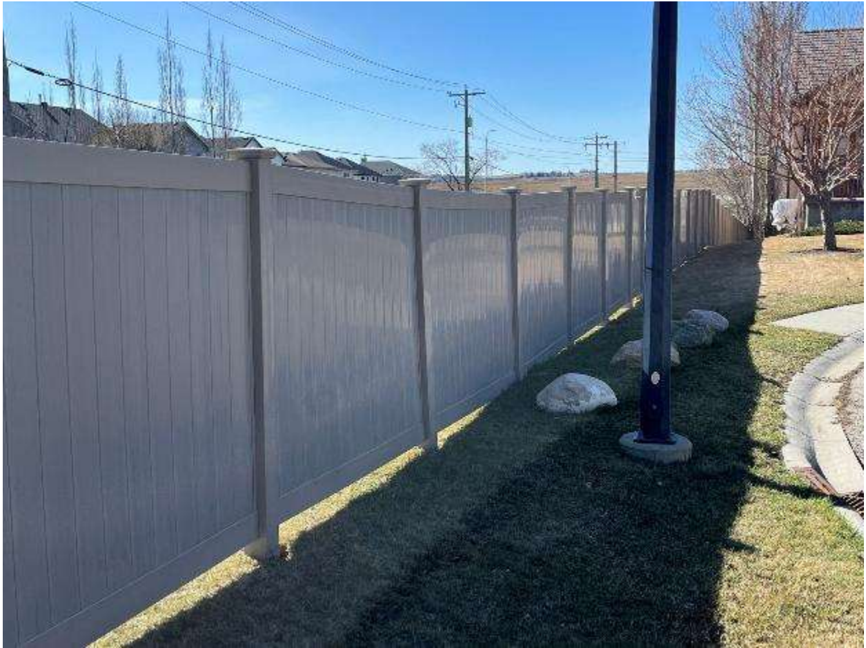
Figure 1 Vinyl fence along 24st, note the air gap at the bottom rail and the structural integrity of the fence
