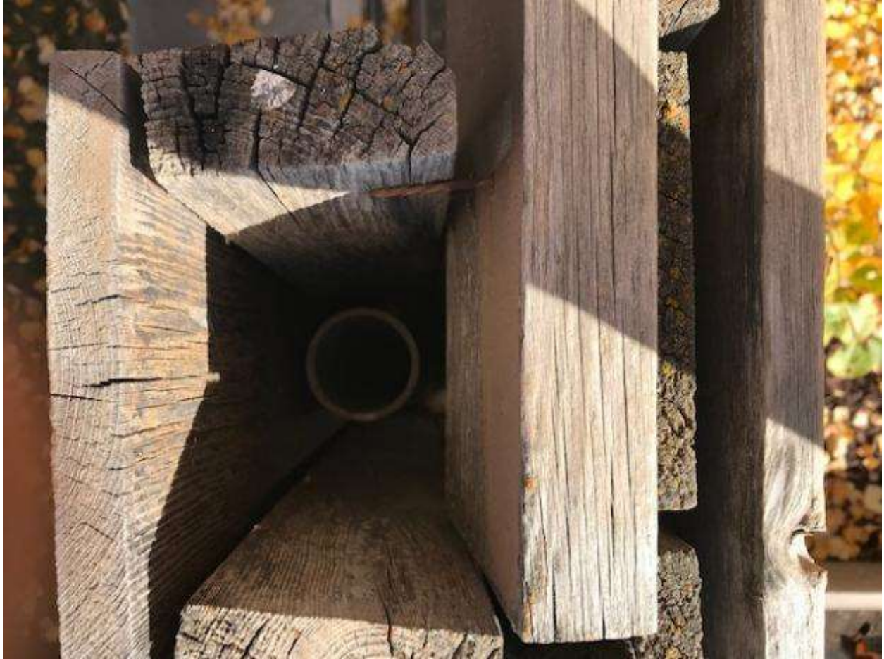
Figure 19 post constructed with wood surrounding a pipe which has contributed to the lean in the fence
