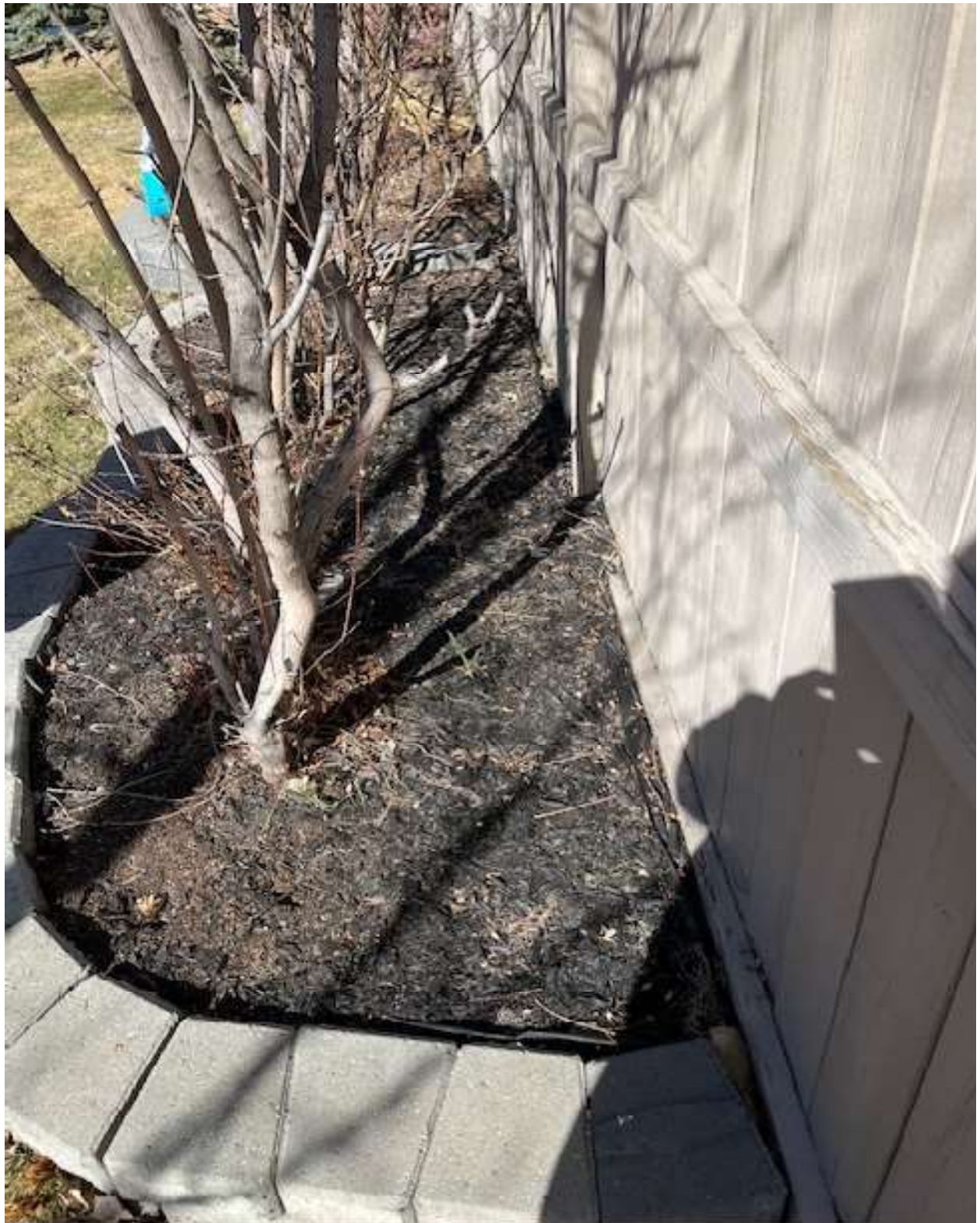
Figure 11 Material next to the fence captures moisture and accelerated deterioration of the wood.
