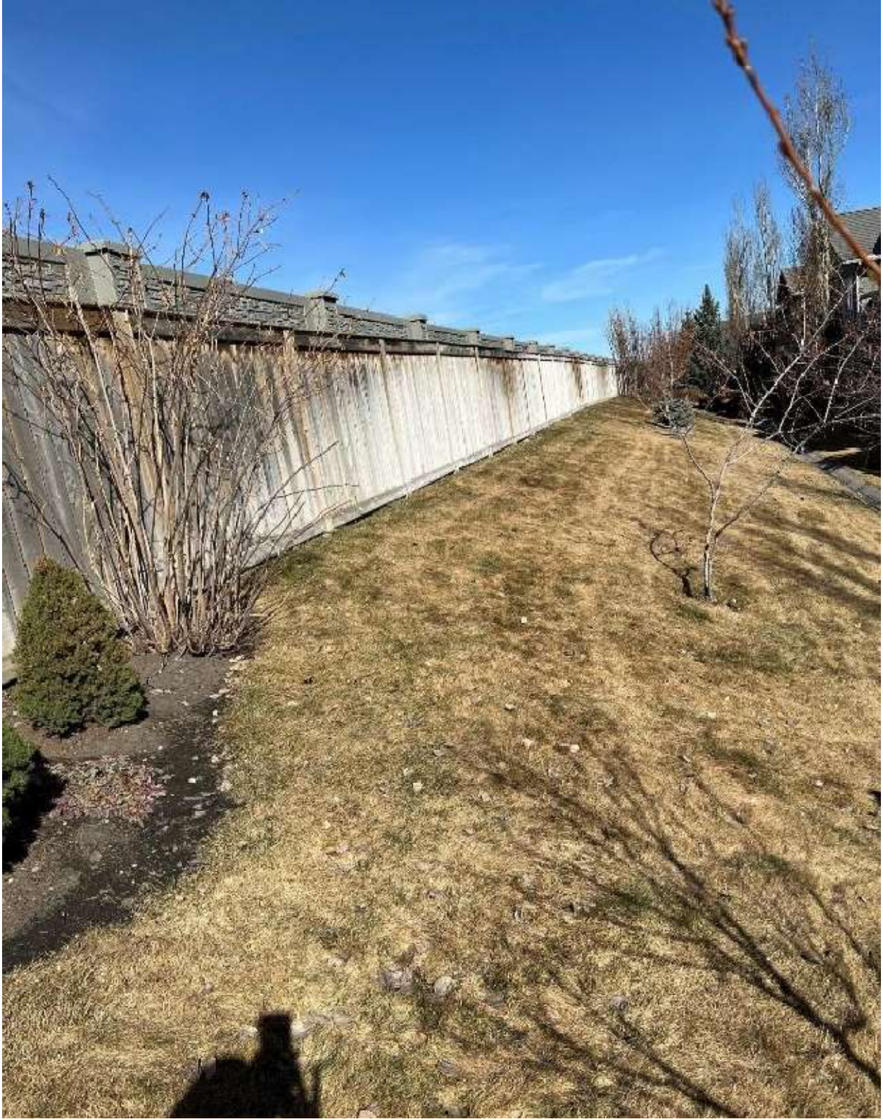
Figure 21 West perimeter fence irrigation sprinkler washed, sun bleached and rustic patina.
