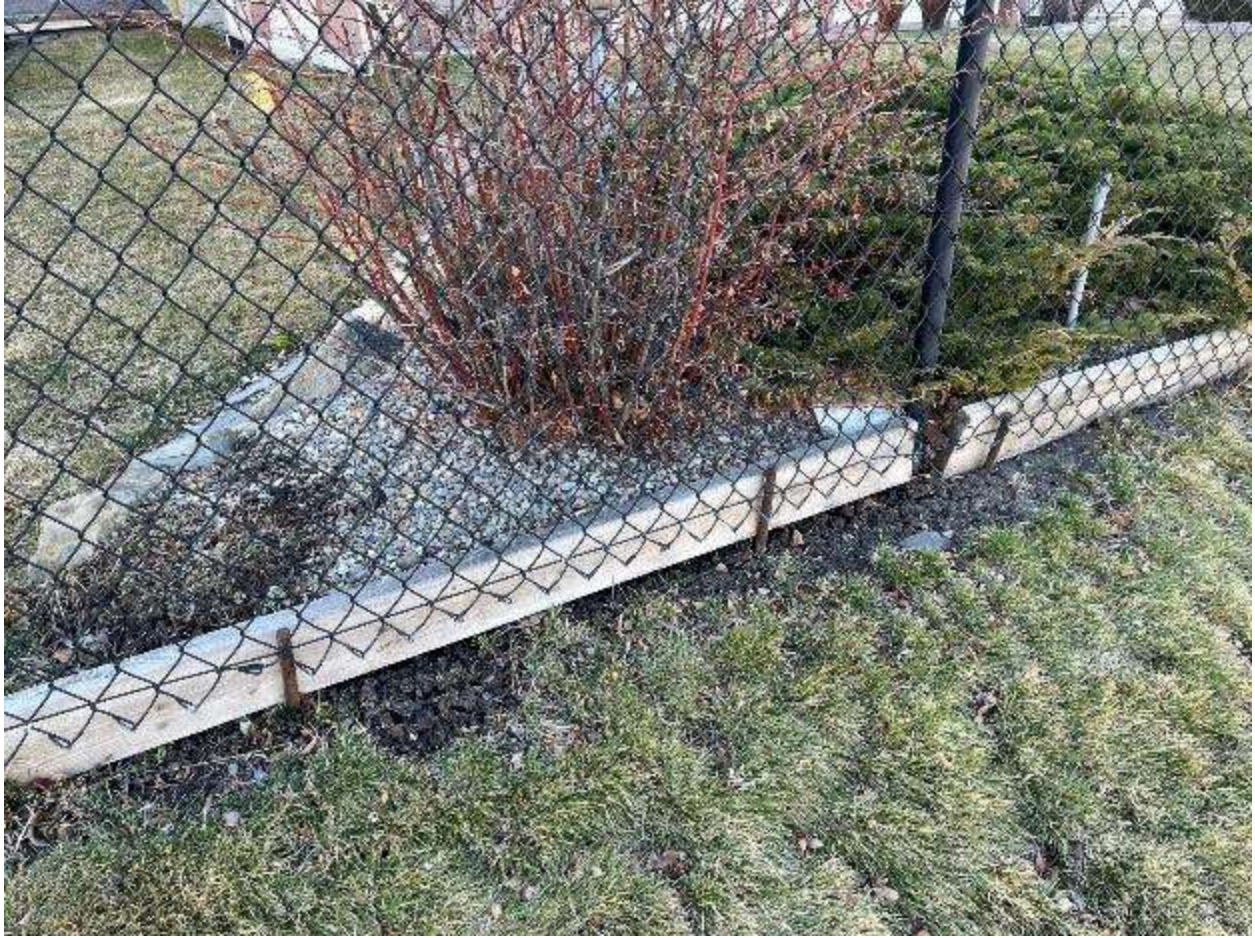
Figure 7 chain link fence with reduced loading on the wire stringer and chain link provided by the board and rebar
