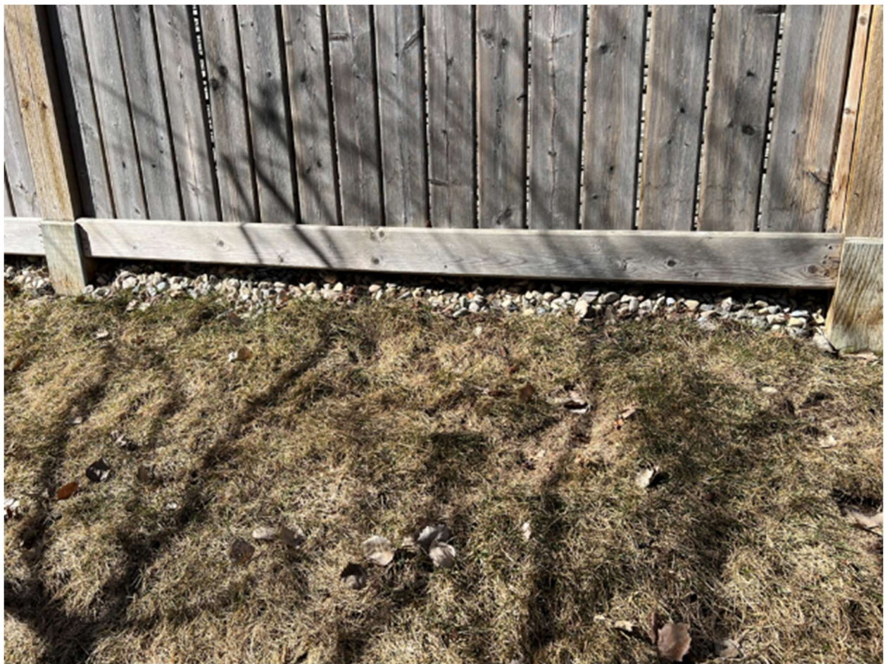
Figure 25 West perimeter fence indicating 3/4 inch plus seeping beneath the bottom rail.
