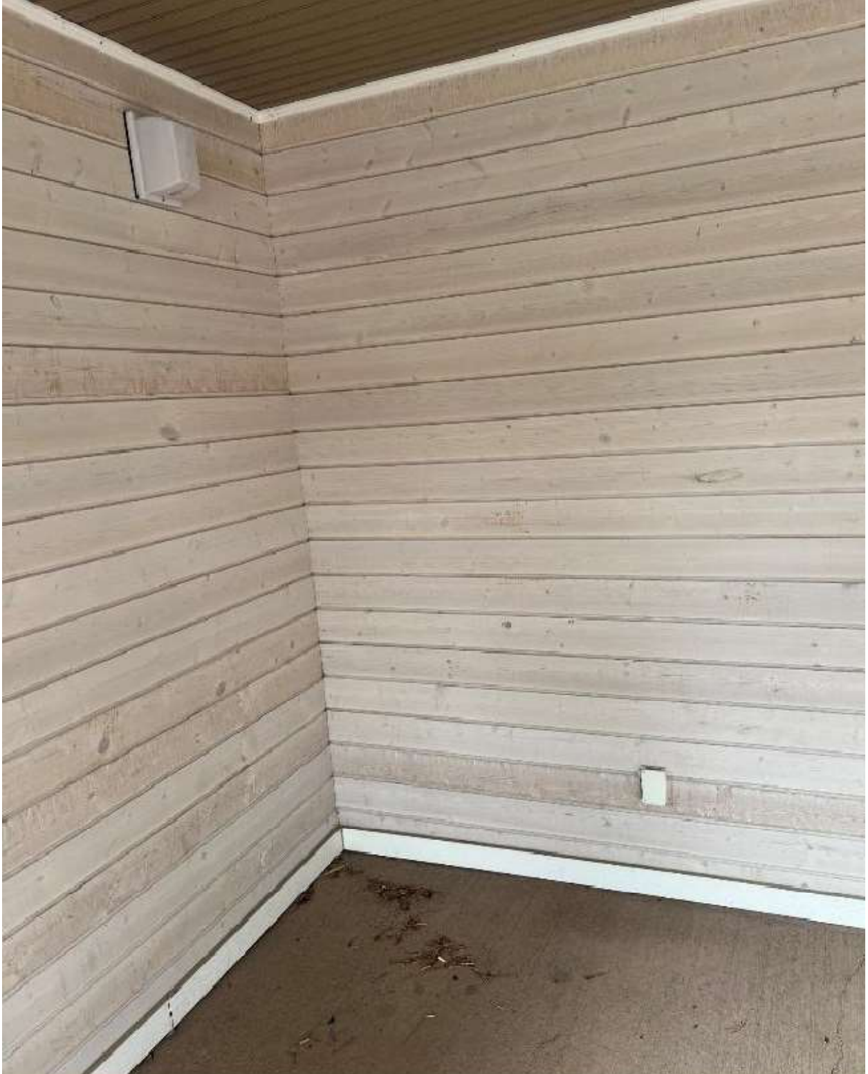
Figure 33 Interior wall of the pavilion indicating the white washed-stained walls.
